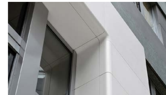
One of the most important features when using HIMACS on a façade is its ability to create round corners.
