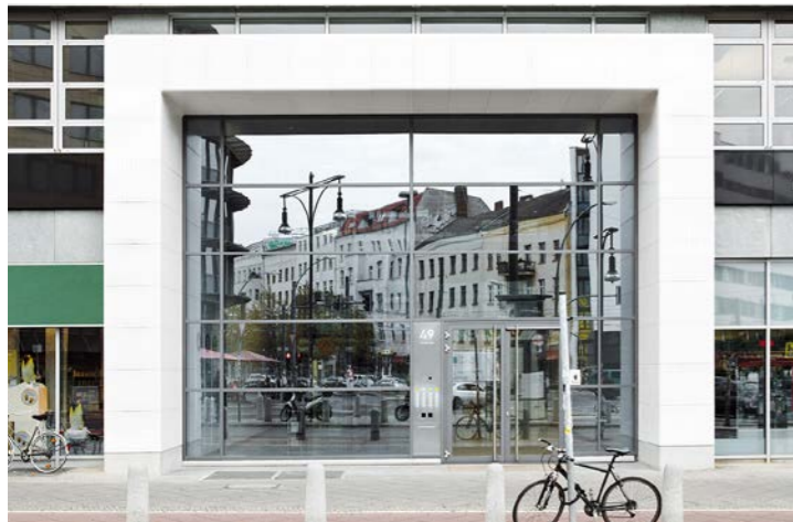
During the day, the lighting technology is invisibly hidden and protected by the robust HIMACS surface.
